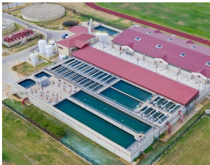
Bud Ervin Water Treatment Plant
